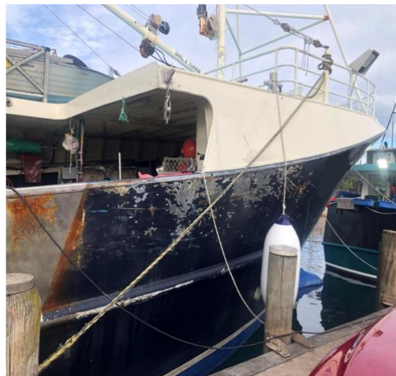
Figure 1.3 Structural damage observed below the gunwale of a tuna longline vessel (blue area) caused by repeated flyback impacts from recoiling weighted gear during hauling operations.
